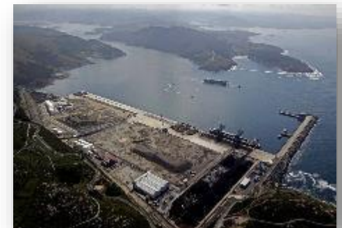
Client: Port Authority of Ferrol (Spain)
