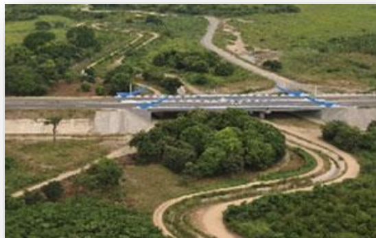
Client: Ministry of Public Works (Ecuador)
