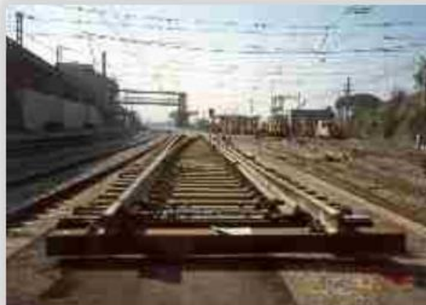
Client: DGF (Spain)
