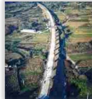
Client: DGF (Spain)
