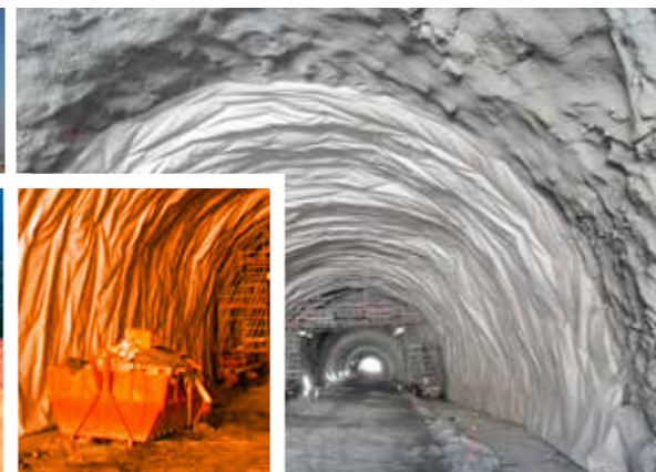
A-7 Motorway, Section: Puntalón – Carchuna, Motril, Spain
