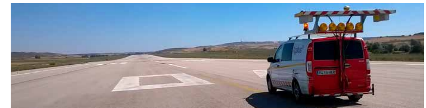
Cracking, macrotexture and roughness measurements with LCMS 3D laser, Burgos Airport, Spain
