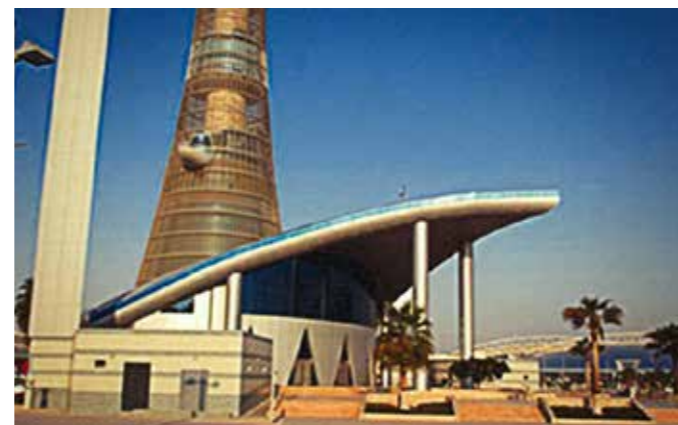
Periodic inspection in the sports complex Aspire (Qatar)
